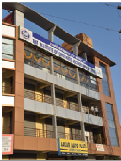
Vapi Branch of ICAI ,Building
